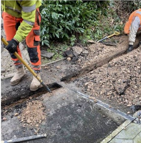
Digging a new trench and tunnelling under the Kerbo Charge channel
